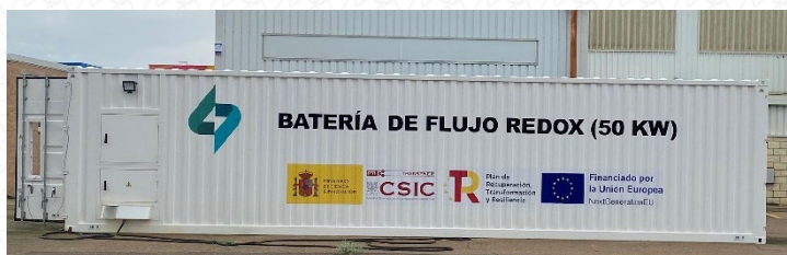
Image: 1 – CSIC containerized 50 kW – 100 kWh Vanadium Flow battery with EPIC POWER bidirectional DC/DC converters
