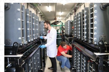
Image: 1 – CSIC containerized 50 kW – 100 kWh Vanadium Flow battery with EPIC POWER bidirectional DC/DC converters
